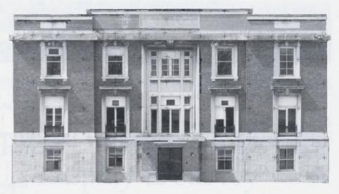
brick and stone, and affords a fine view of both the Canadian and American Falls. It houses office space and machine shops, with underground communication and electric cables to the Niagara transformer station.
